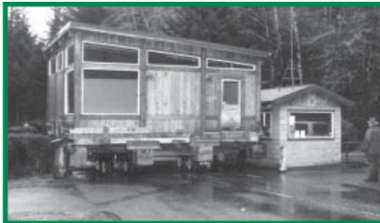
Tight fit at Sunset Campground
