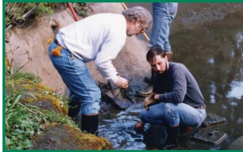
Gregg (L) and BLM volunteer work on pond drain in 1995.
