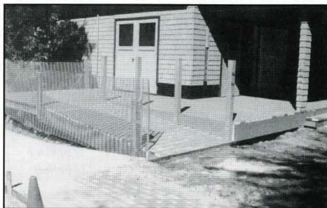
Visitors can look forward to a new porch, ramp, and walkway at the back of the Garden House. Also, the house has been rewired, new heaters have been installed, and Keith Ott has replaced all of the baseboards, which volunteers will put the finishing touches on.
