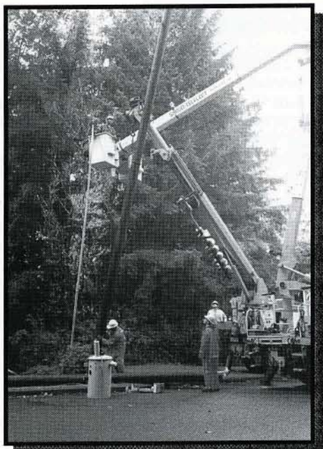
Pacific Power sets final pole in a massive project to upgrade power from Sunset Bay to Shore Acres.
