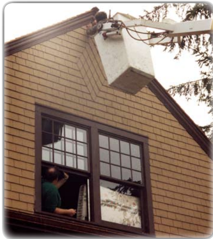
In the Garden House window, Park Manager Andy LaTomme offers advice to Ranger Frank Eckley in the lift bucket at the peak. The lift truck project was filling woodpecker holes in the trim and siding. The plastic was over the porch to protect a non-skid stair-tread paint while it dried.
