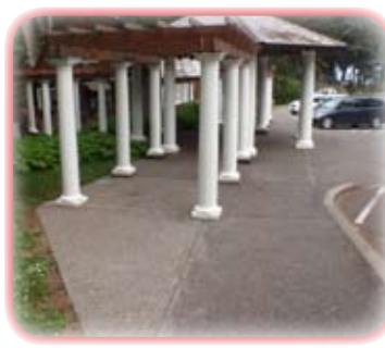
Two aggregate walkways (L) replace asphalt near the Greenhouse with two new aggregate sections added at the entrance.
