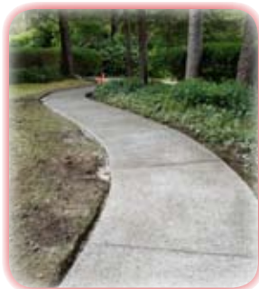
Two aggregate walkways (L) replace asphalt near the Greenhouse with two new aggregate sections added at the entrance.
