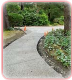
Two aggregate walkways (L) replace asphalt near the Greenhouse with two new aggregate sections added at the entrance.
