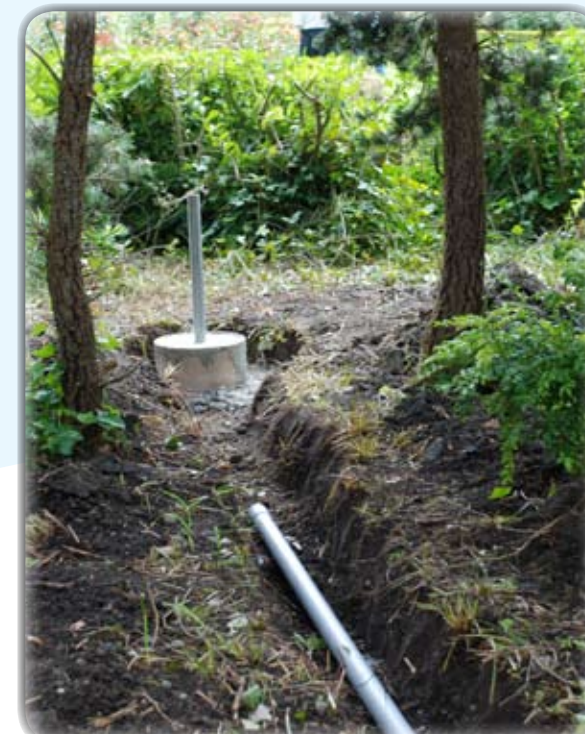
BASE FOR WILD BLUE SATELLITE DISH NEAR THE NORTHWEST GARDEN.
