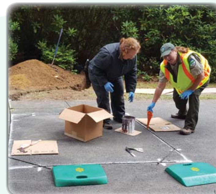
Park Rangers Pam Stevens and Ellie Kinney-Martial install new traffic counter loop at Shore Acres.
